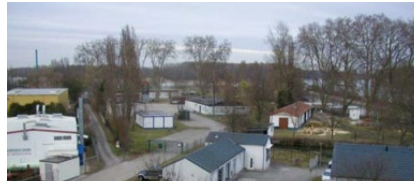
Buildings in the floodplain
