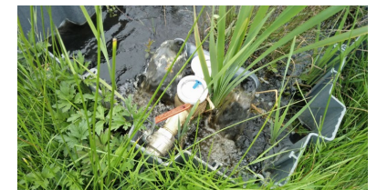
Re-pumping when the water level drops. The water meter measures the amount of water supplied. © A. Bartel
