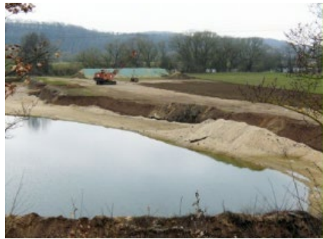
Excavated water body
